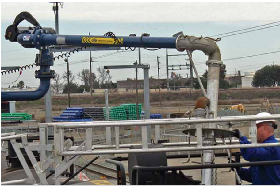
The terminal manager at NuStar's Stockton facility, says he can't be more pleased with the new loading system
