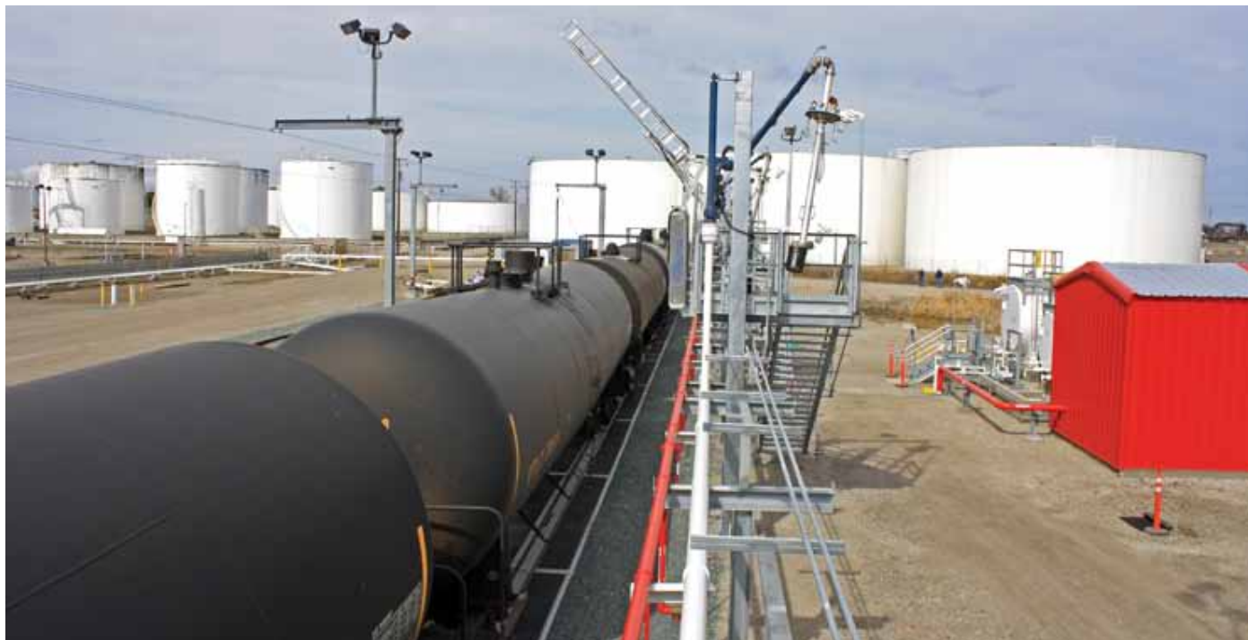
The Stockton terminal's new rail siding features six loading platforms
